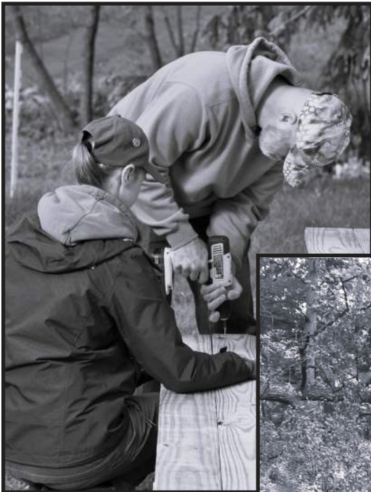
Park Day volunteers build new picnic tables.
