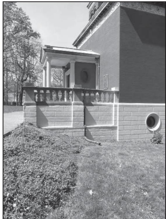
Stucco around the base of the Study was recently repaired thanks to a generous grant from the Tippecanoe Arts Federation. The above photos show the badly damaged stucco (*left*) and the repaired stucco (*right*).
