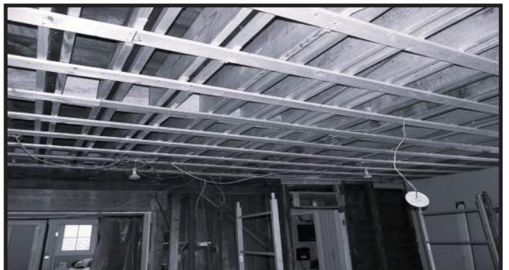
Installed firring strips to level ceiling.
