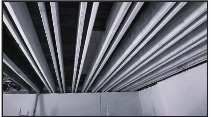
Original joists sistered with new joists.
