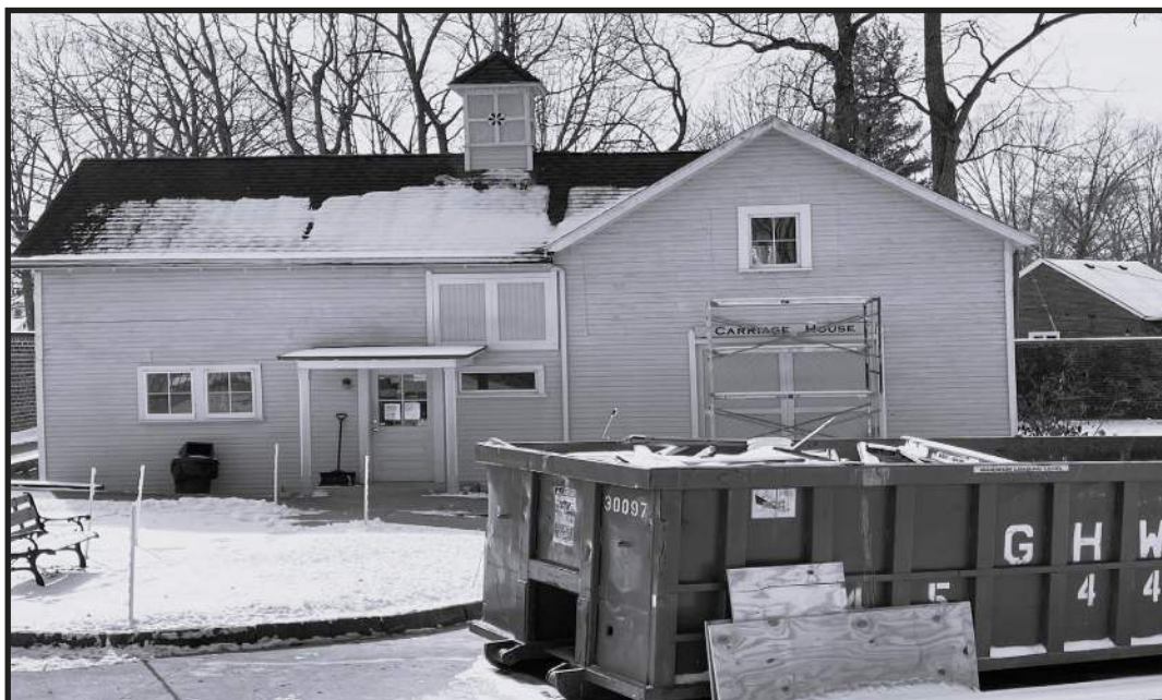
Winter Carriage House construction site.
