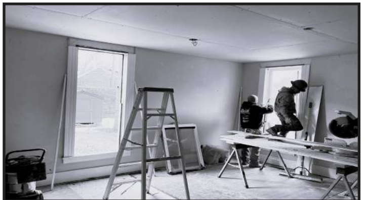
Restoring the windows.
