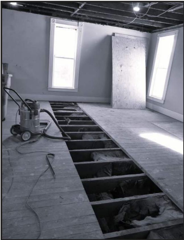
Crawlspace access to repair foundation piers.
